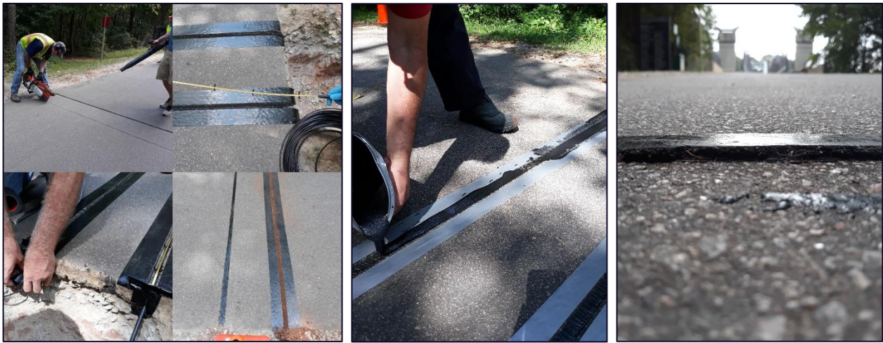
Figure 6. Initial Installation (left), Applying Additional Resin (center), and Final Pressure Pad Height (right)
