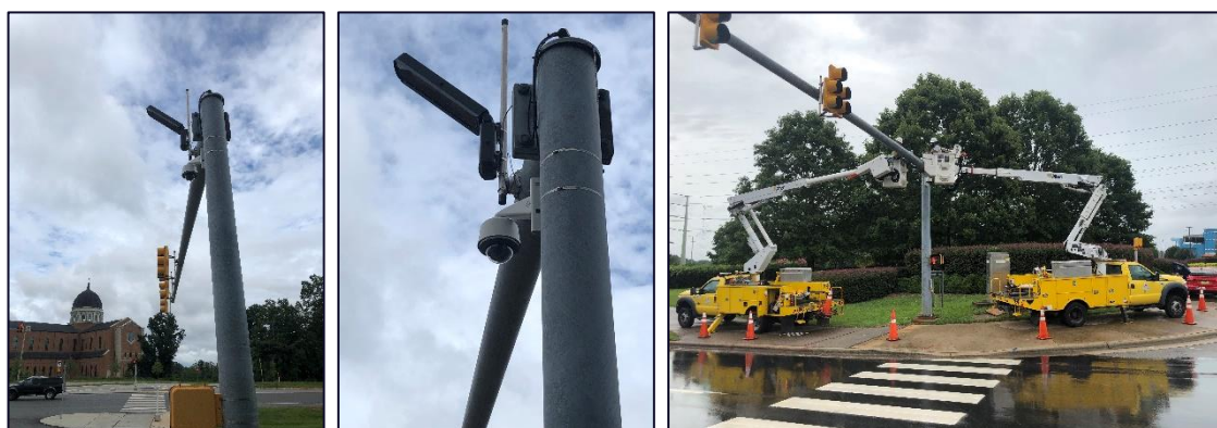
Figure 12. CITIX 3D Installation on the Horizontal Mast Arm of a Traffic Signal
