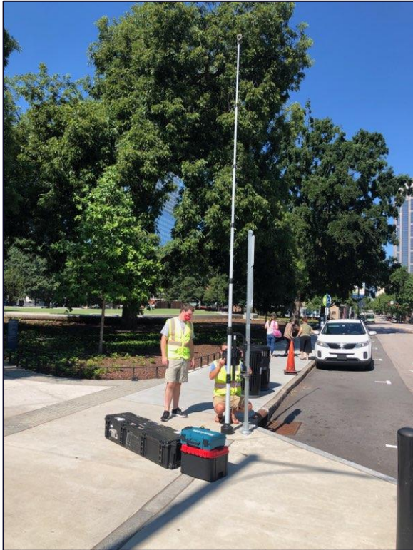
Figure 10. Miovision Scout Installation on a Parking Sign
